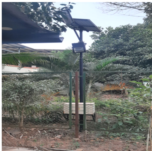
Figure 7.5.6: IoT Based Solar Powered Street Light control and monitoring
